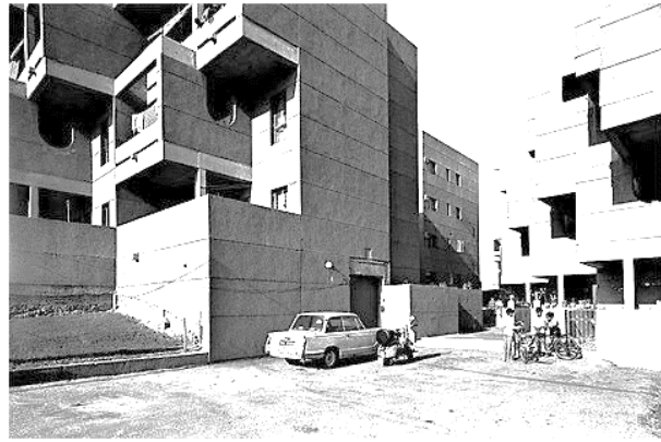
Figure 14: Yamuna Apartments (Source: The Design Group - Yamuna Apartments (1981), Alaknanda in southeast Delhi)
